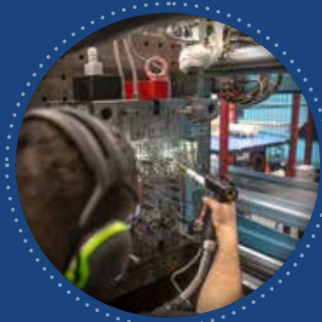
Replacement of Worn Components
